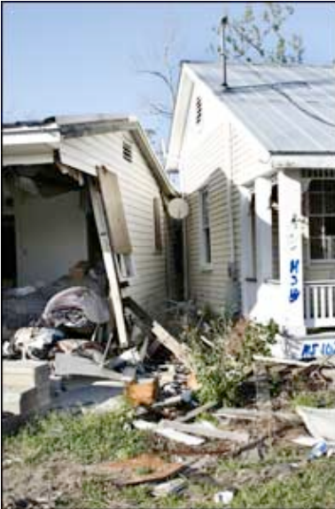
Two homes that were pushed into one another during the tidal surge. Many homes have not been touched since the hurricane; the bedroom contents of the home on the left are still present.
