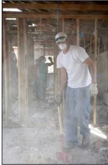
NAU student Mike Davis scoops up debris created from tearing out the interior of this Mississippi home.
