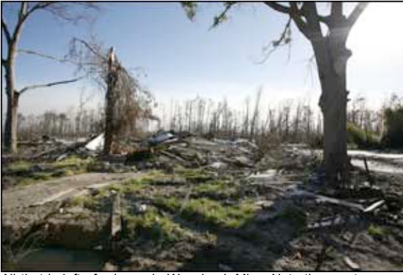
All that is left of a home in Waveland, Miss. Note the empty foundations surrounding this property. There are almost no remaining structures in the neighborhood.
